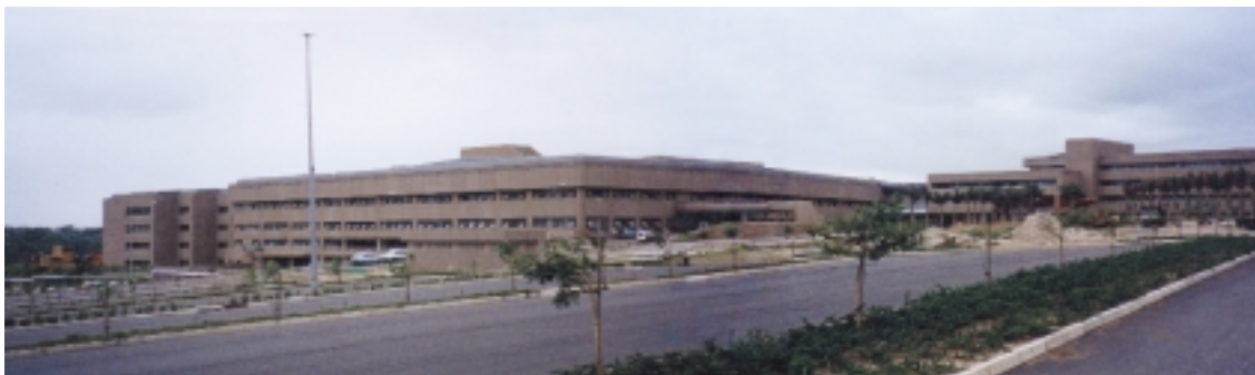
The Inkosi Albert Luthuli Central Hospital fitted with a tube-mail communications system.
